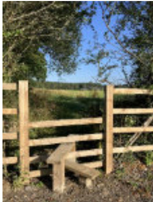
Newly installed stile on FP
