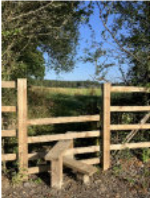
Newly installed stile on FP
